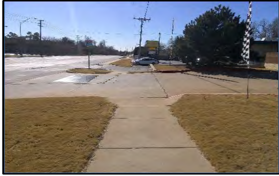
Corner 1 No Ramp (1z)
