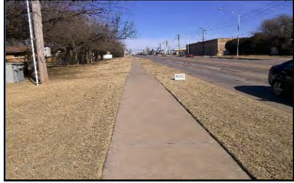
Corner 4 No Ramp (4z)
