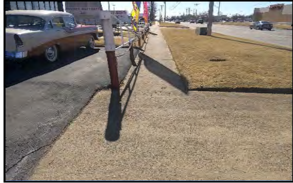
Corner 3 No Ramp (3z)
