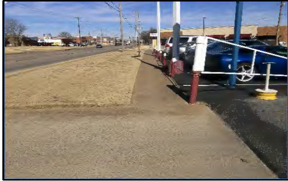
Corner 2 No Ramp (2z)
