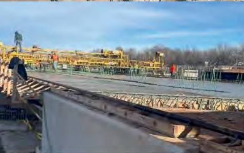
James Garner Ave. Bridge Construction
