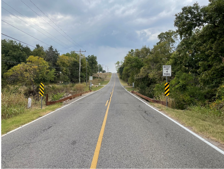
Roadway view with load posting of 4 tons, looking south
