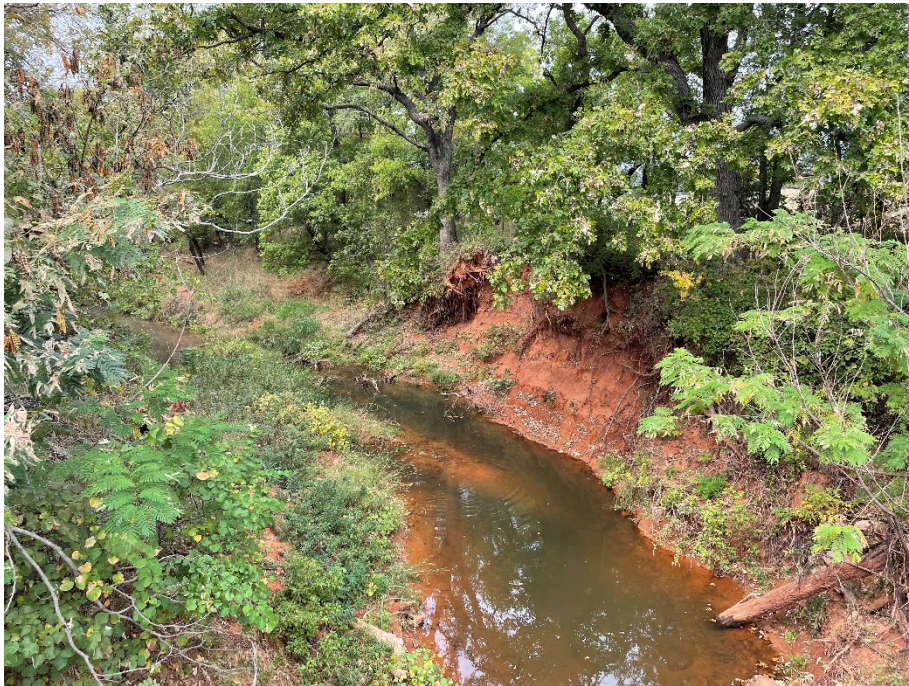
Channel view, looking west
