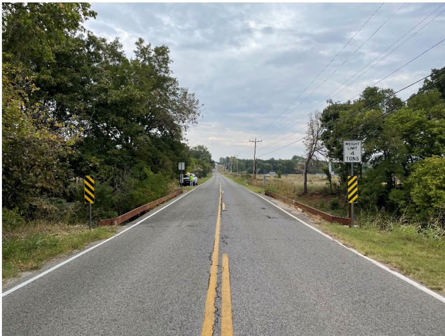
Roadway view with load posting of 4 tons, looking north
