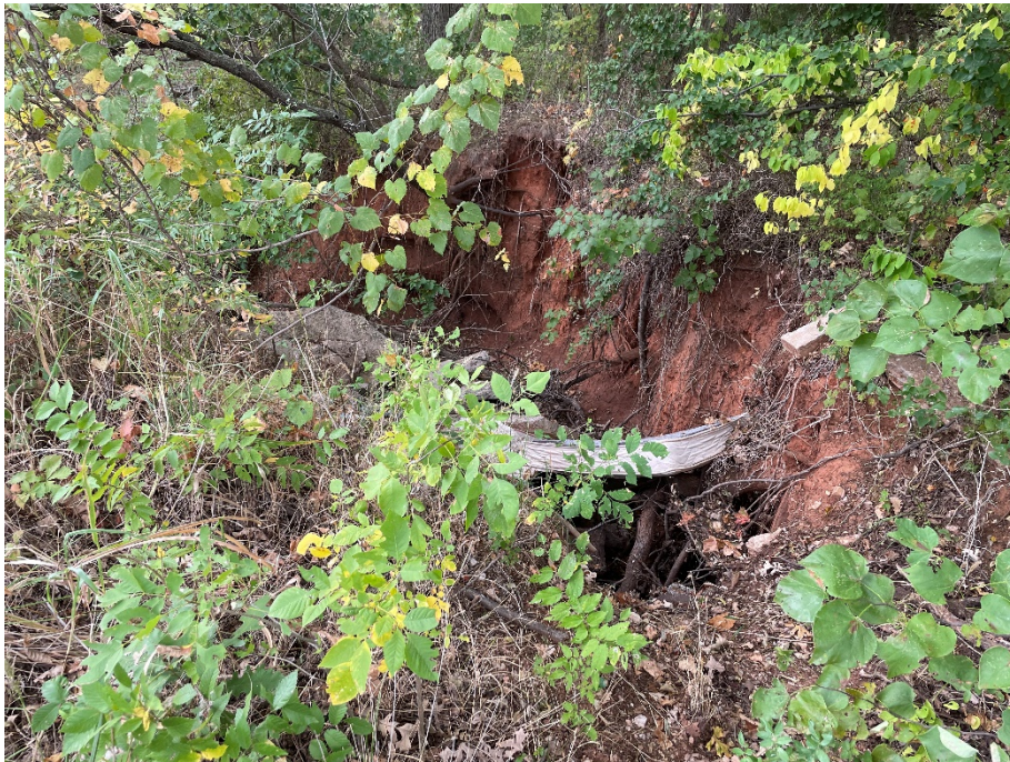
Northwest ditch erosion
