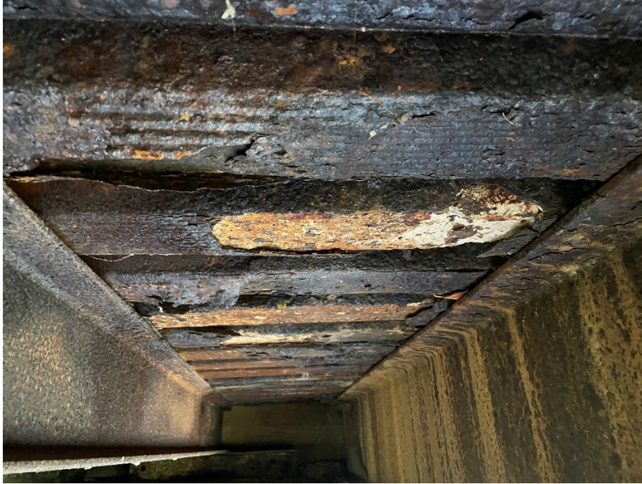
Typical view of SIP forms
