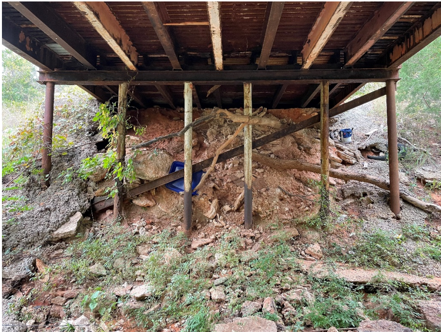
Typical condition of superstructure, looking at northside of pier 1
