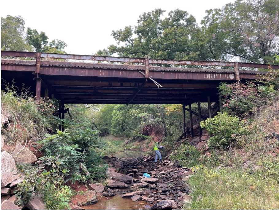
Elevation view, looking west
