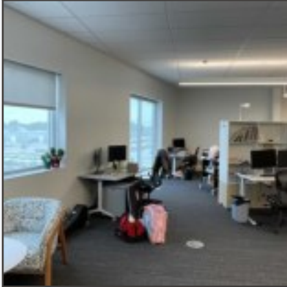
Area setup prior to containment
