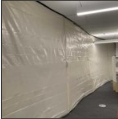
Containment setup in progress
