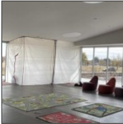
Containment setup in progress
