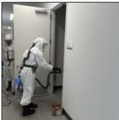
Second Floor - Main Area: 11/17/23 - Fogging
