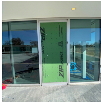
16. First Floor - 149 Storytime: Window Removal for Negative Air Ducts
