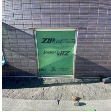
15. First Floor bay windows: Zip sheathing install on East Window
