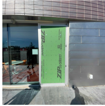
15. First Floor bay windows: Zip sheathing install on East Window
