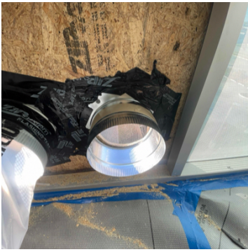
48. 305 Pioneer: Signs of Possible Water Intrusion
