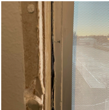
63. 201A Staff Only: Potential Source of Water Intrusion Daylight is visible through a gap in the tall window frame.
