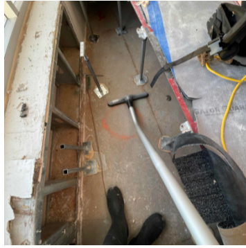
63. 201A Staff Only: Potential Source of Water Intrusion Daylight is visible through a gap in the tall window frame.
