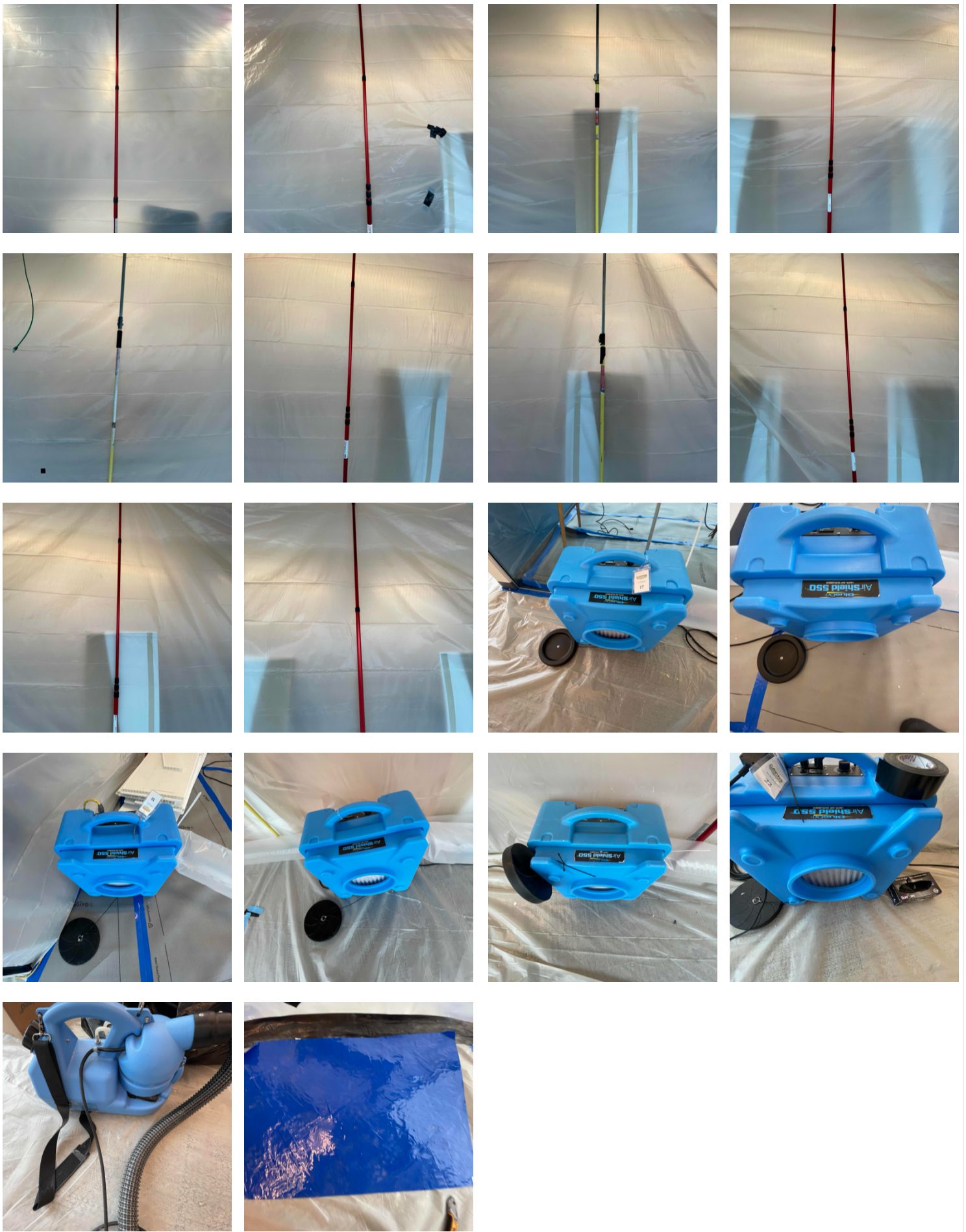
10. Second Floor - Southeast Corner: Filter Change
