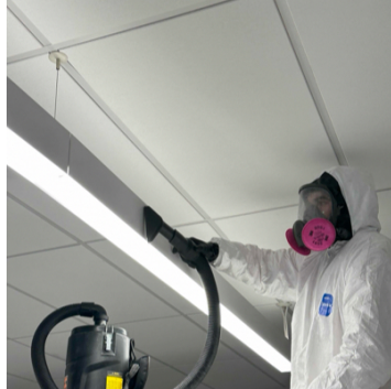
43. SO 115: Phase 2 cleaning Hepa vacuum ceiling, walls, & floors. Wipe ceiling, walls, & floors
