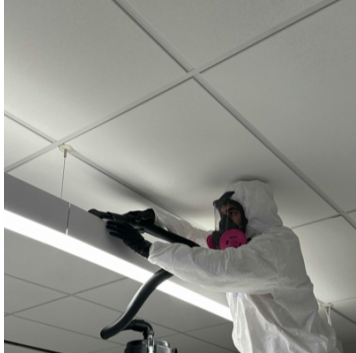
43. SO 115: Phase 2 cleaning Hepa vacuum ceiling, walls, & floors. Wipe ceiling, walls, & floors
