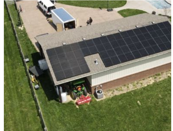
Outbuildings Providing Power
