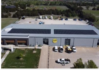
Pella Windows & Doors Showroom & Warehouse
