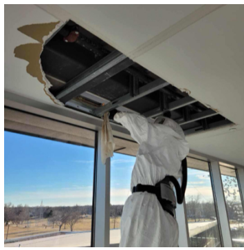
41. Fogging- All common areas of all three floors have been fogged as a preventative measure due to moisture entering building from recent rain fall.
