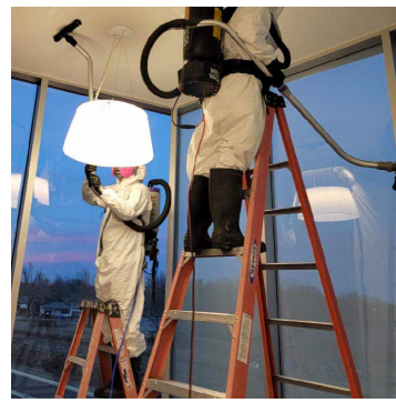
41. Fogging- All common areas of all three floors have been fogged as a preventative measure due to moisture entering building from recent rain fall.
