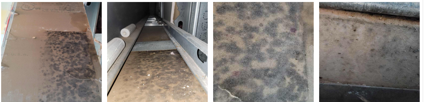
18. Second Floor - Southeast Corner: Study Room Remediation Microbial growth was found on back side of ceiling drywall
