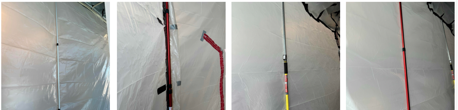
10. Second Floor - Southeast Corner: Equipment 22 - Zip Posts 6 - Air Scrubbers 1 - 50' Extension Cord
