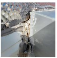
3. Second Floor - Southeast Corner: Water Testing Water intrusion from soffit area at top of corner windows Water intrusion from roof/window connection
