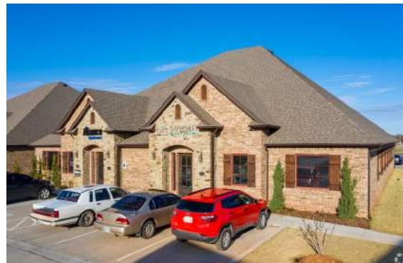
GulfTex Energy IV, LP Built: 2017 Vacancy: 50.0% Size: 3,450 SF Asking Rent: $20.00 PSF
