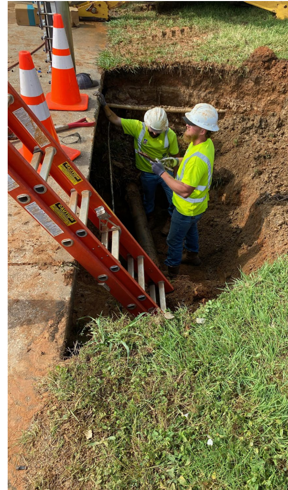
Line Maintenance workers repair a water pipe in June 2023.
