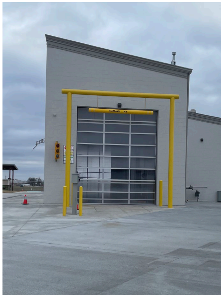
North Base Vehicle Wash Facility exterior and interior
