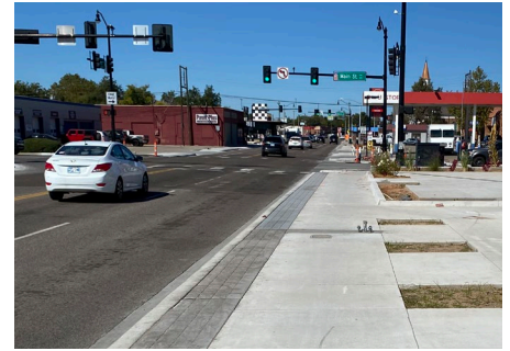
Completed sidewalk and planters near Porter Avenue and Main Street
